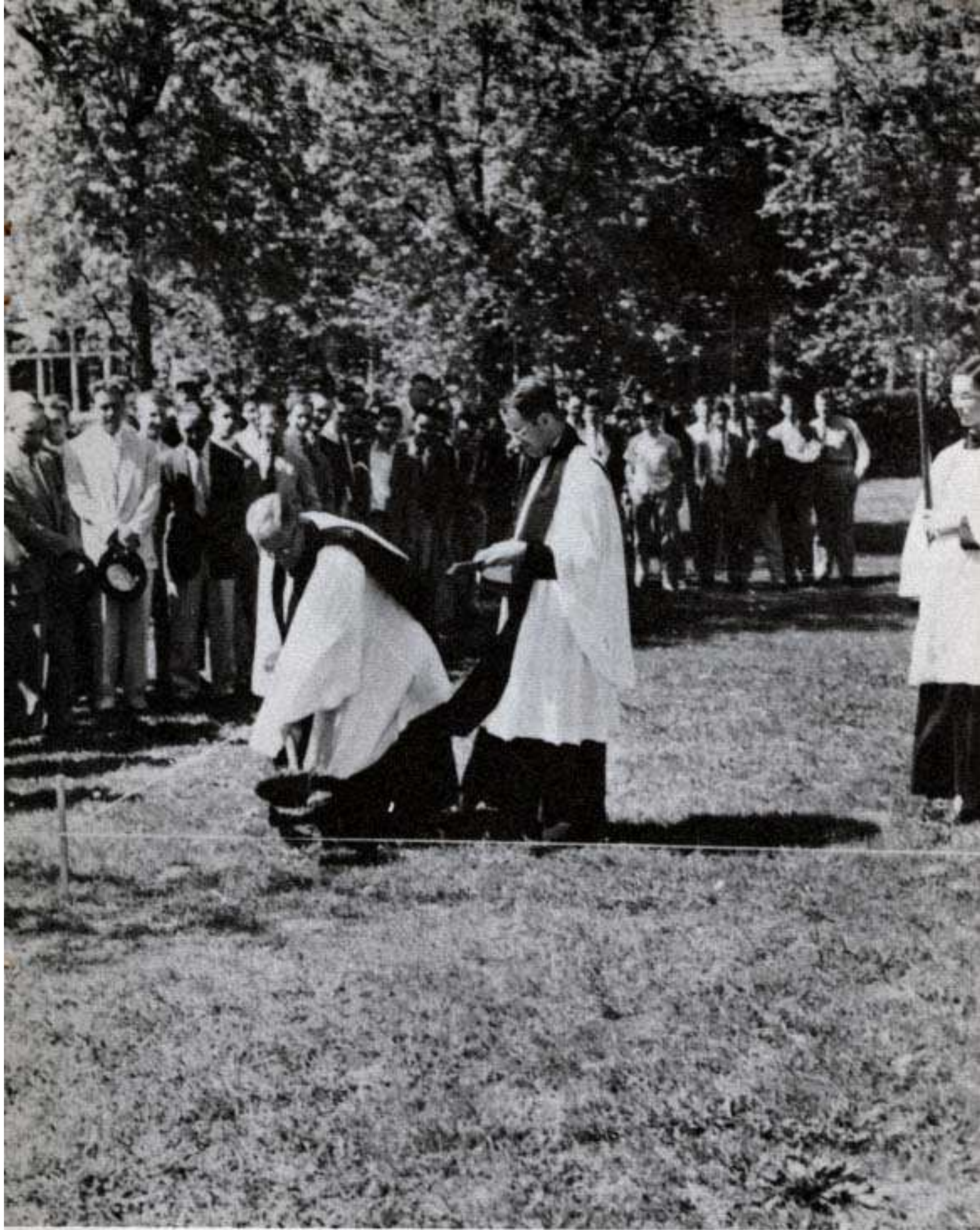
Dr. Pell breaks ground for the final addition to the Main Building and for the Irene du Pont Library, May 1955.
